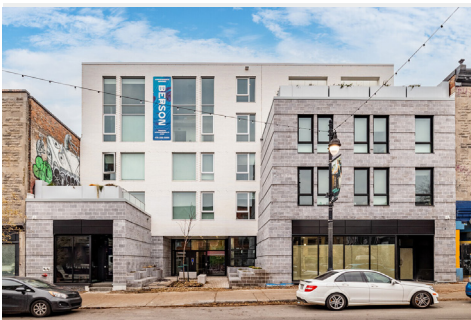
Façade de Berson - Berson Facade
