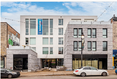
Façade de Berson - Berson Facade
